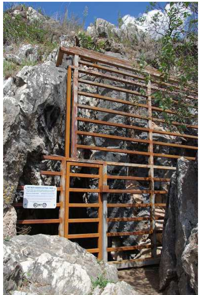
Above: The first day of work in January 2019 to replace vertical rods with horizontal square-section tube
